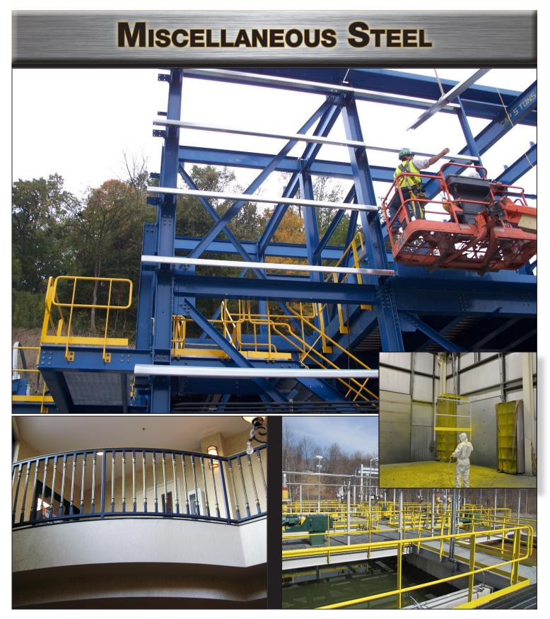
All work is visually inspected by Certified Welding Inspectors and recorded as per AISC and AWS codes. Our paint facilities are complete with Wheelabrator and shot blast rooms. Surface preparation of steel and painting are checked by the Lincoln Contracting quality control team and surface profile and paint millage is recorded. Rely on Lincoln Contracting to provide you with exceptional quality and customer service.
