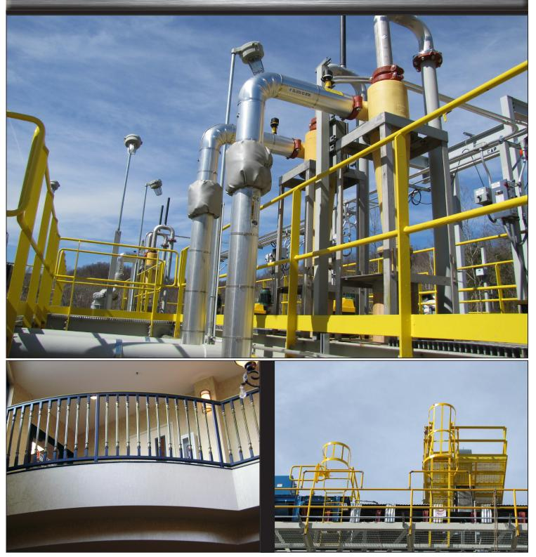
All work is visually inspected by Certified Welding Inspectors and recorded as per AISC and AWS codes. Our paint facilities are complete with Wheelabrator and shot blast rooms. Surface preparation of steel and painting are checked by the Lincoln Contracting quality control team and surface profile and paint millage is recorded. Rely on Lincoln Contracting to provide you with exceptional quality and customer service.
